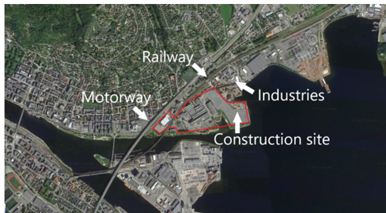
Figure 1: Location A, the construction site for the new hospital in Drammen, Norway [5].
